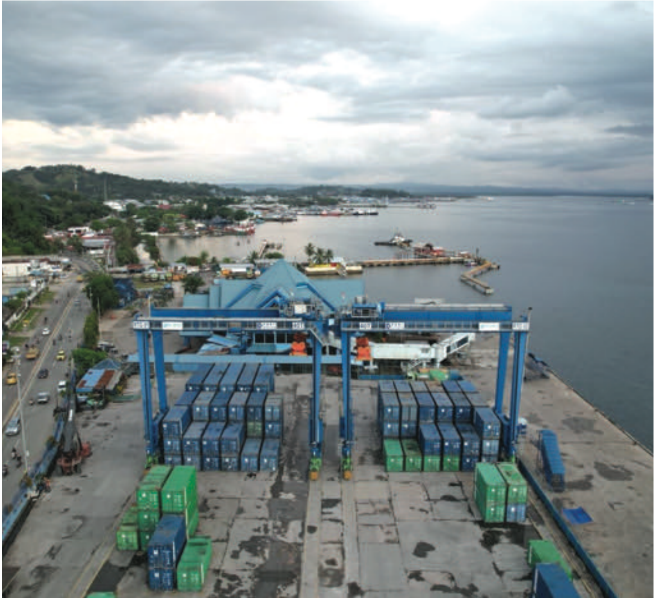
Keterangan : Pelabuhan Peti Kemas, Port of Sorong di Kota Sorong / Caption: Container Port, Port of Sorong in Sorong City.
